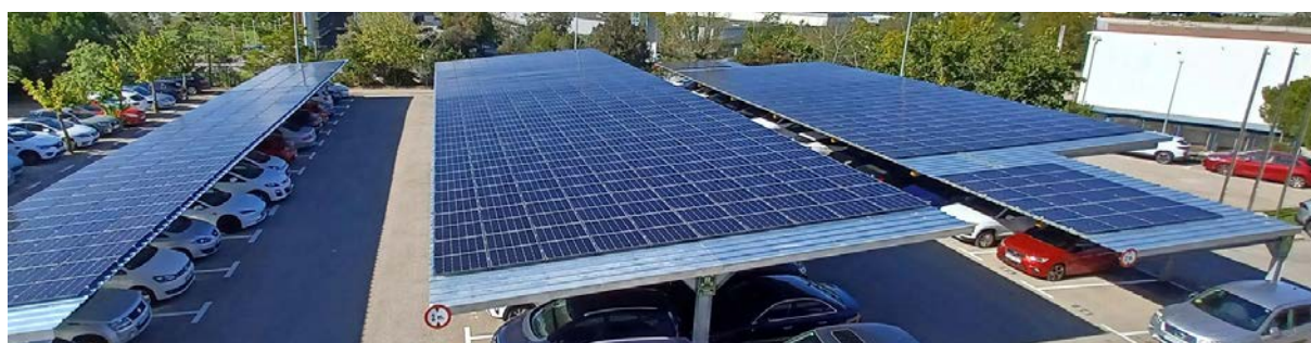
Installation of a 187 kWp photovoltaic system located at the Sportium and B2B headquarters in Sant Cugat (Barcelona)
